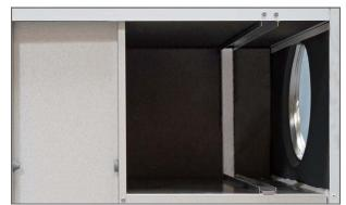
5. The new filter is placed in the marked tracks and the door is closed again.
