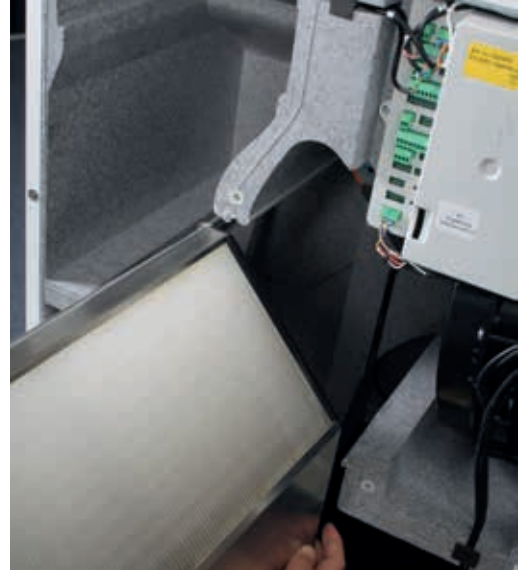
Remove counterflow heat exchanger
