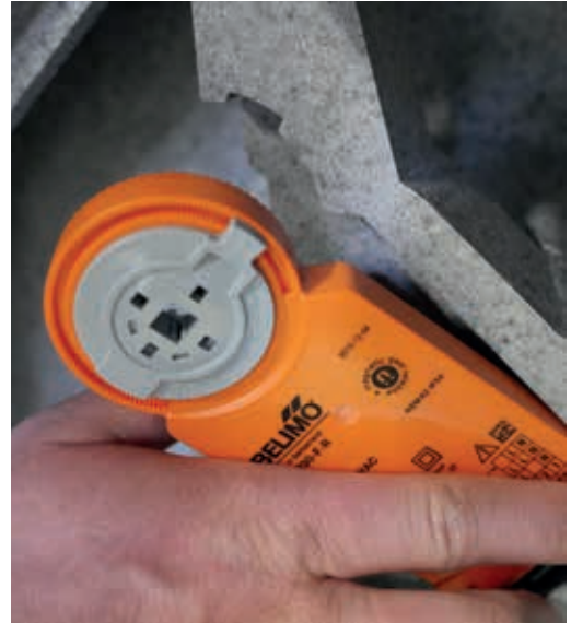
Remove bypass actuator
