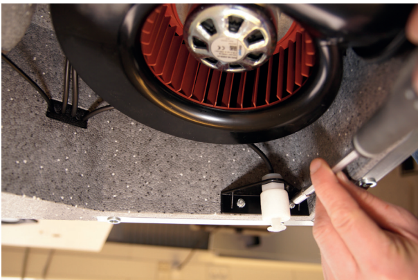
Remove condensate drain switch
